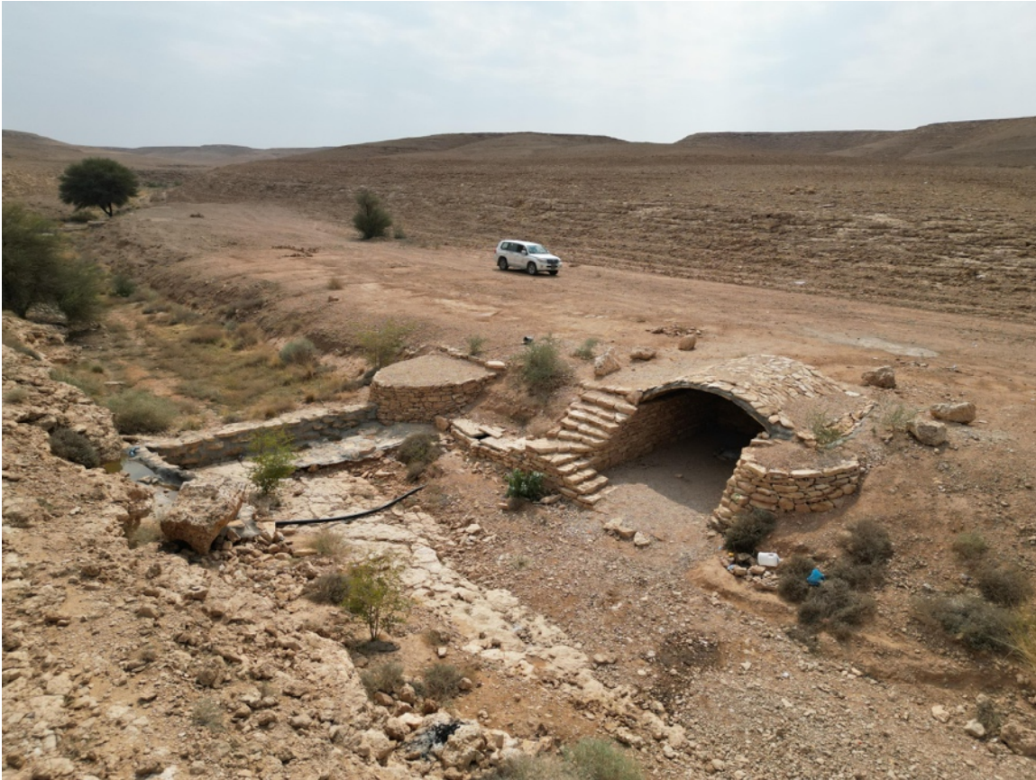
Figure 4. Cross-wadi wall, (50 cm high), with a cave for tourists to rest in the shade, in Thadiq National Park (© Éric Lacroix)
