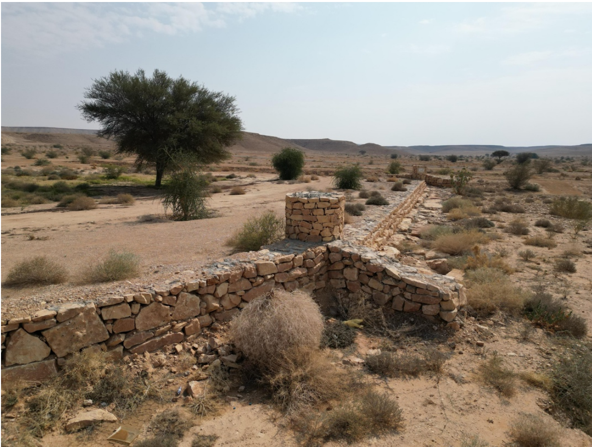
Figure 2. Cross-wadi wall with tower and wings with a < 1 meter wall in Thadiq National Park (© Éric Lacroix)
